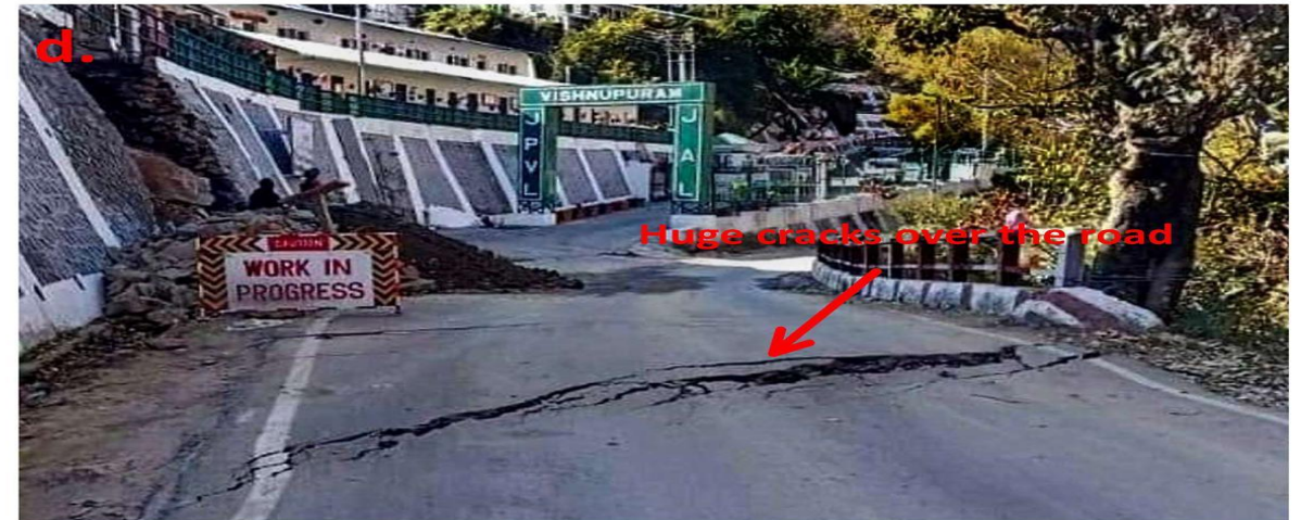
Figure 3: Ground truth validation — (a,b) structural cracks in buildings, (c) wall collapse, (d) road deformation. All detected by InSAR before visible damage appeared.
